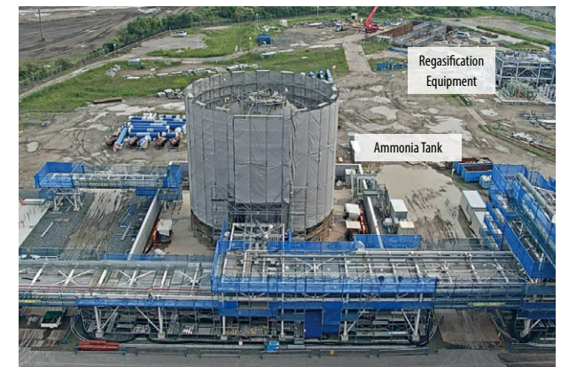
Construction Progressing on Ammonia Demonstration Test Facility at Hekinan Thermal Power Station
